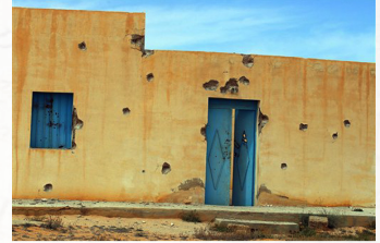
The wall of a house bears the signs of fighting as Tunisian soldiers search for attackers still at large in the outskirts of Ben Gardane, southern Tunisia, Tuesday, March 8, 2016. (Source: AP Photo.)
