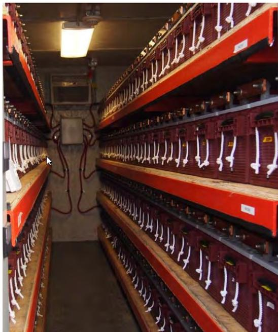
**Figure 5.9 Battery bank for mini-grid in Les Anglais, Haiti.**
